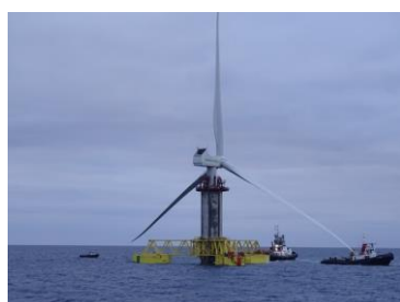
Figure 243. Offshore marine wind turbine in Gran Canaria (photo from PLOCAN, www.plocan.eu )
